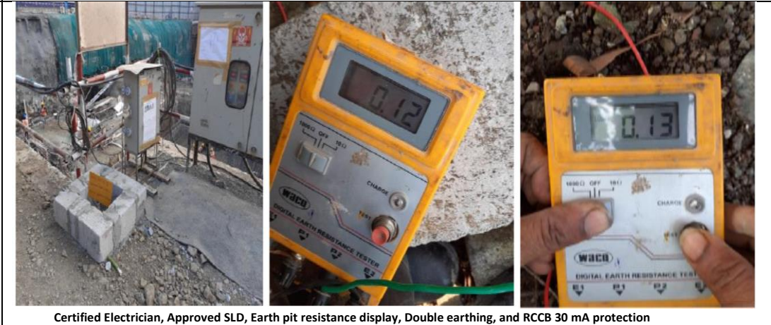
Certified Electrician, Approved SLD, Earth pit resistance display, Double earthing, and RCCB 30 mA protection
